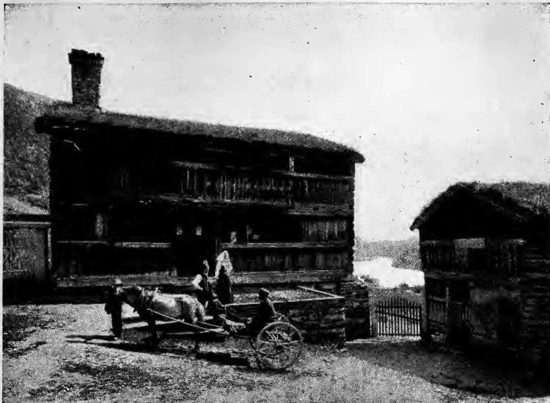
OLD POSTING STATION, WITH CARIOLE. AASOREN, GUDBRANDSDALEN. The architecture is from the sixteenth century.
